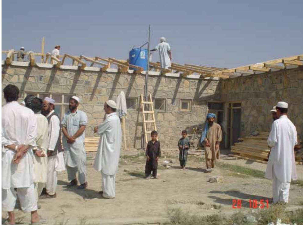
A clinic building under repair in Lakan District, Khost Province
