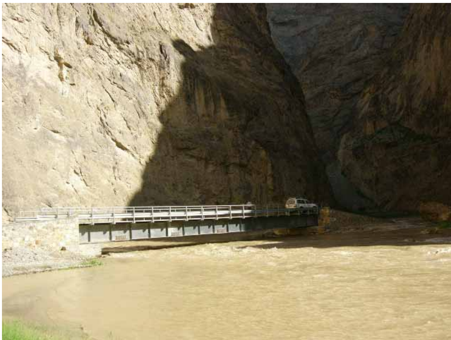
Bailey Bridge in Kunda Sang, Bamyan, constructed by USAID-PRT Project under NABDP-DEX
