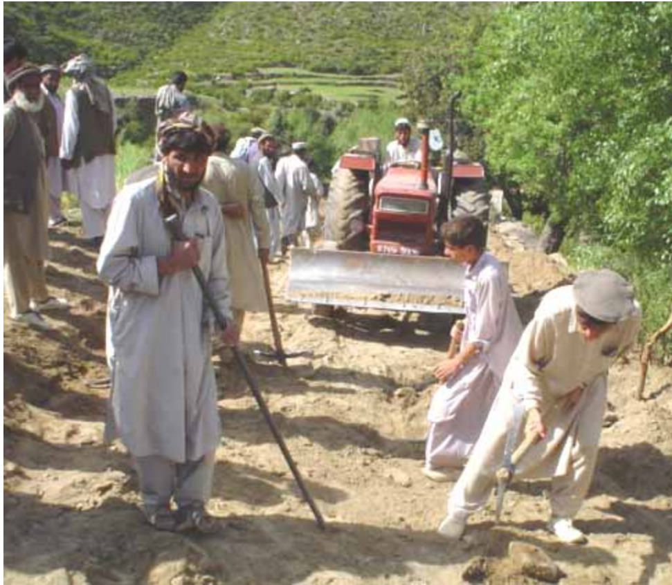
A road construction site in Paktika
