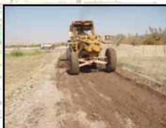
Construction of Road in Uruzgan Province - 2008
