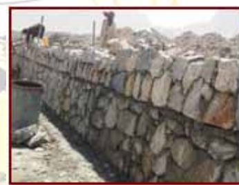
Retaining Wall - Arghandab District Kandahar - 2007
